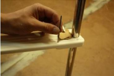
12. Remove the tread as before and repeat the drilling process.
